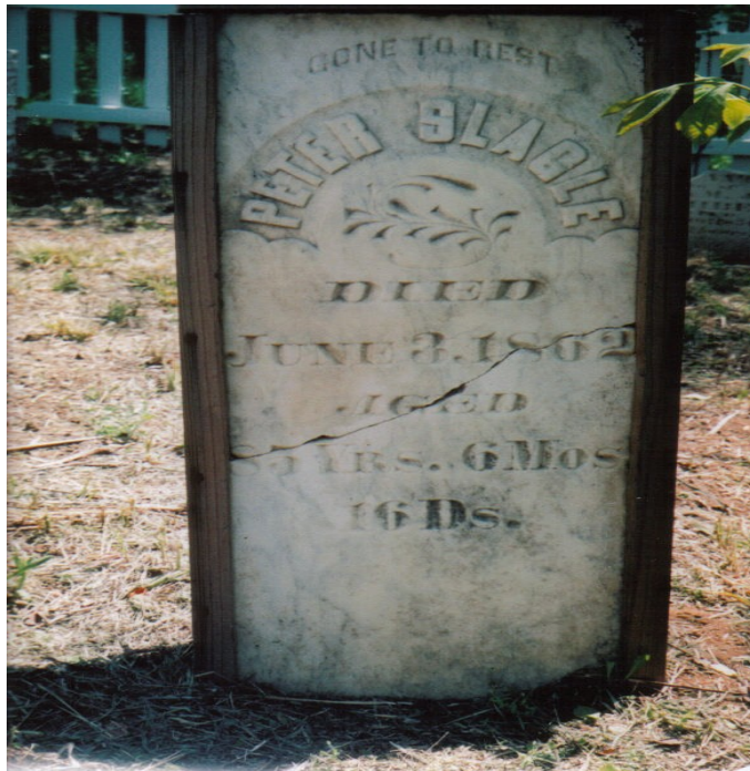
The stone of Peter Slagle Died June 08, 1863 aged 83 yr 6 months 16 days. This stone was found broken and was set in a pressure treated wood frame
